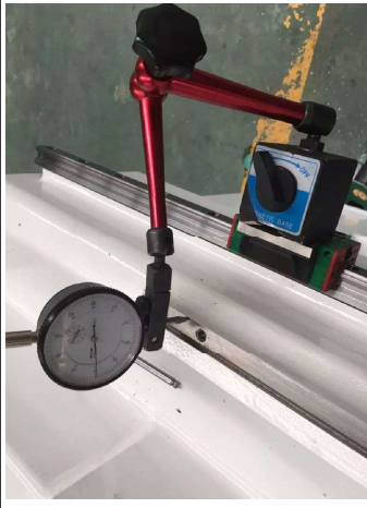
5. Machine rack and rails installed based on the dial indicator, table frame based on the marble gradienter. This quality engineering and workmanship result in smooth precision cutting.
